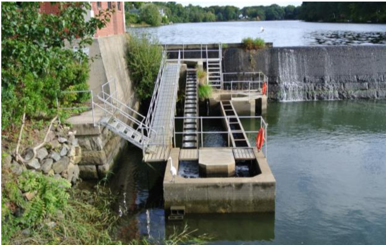
LISFF-funded fishway and access walk at Mianus River Pond.
