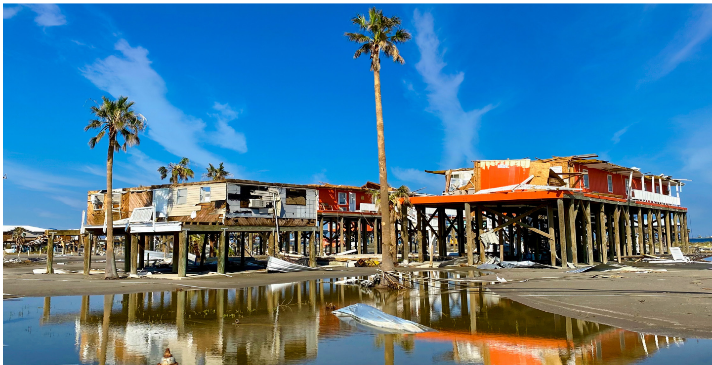
Damage from Hurricane Ida in Grand Isle, Louisiana
