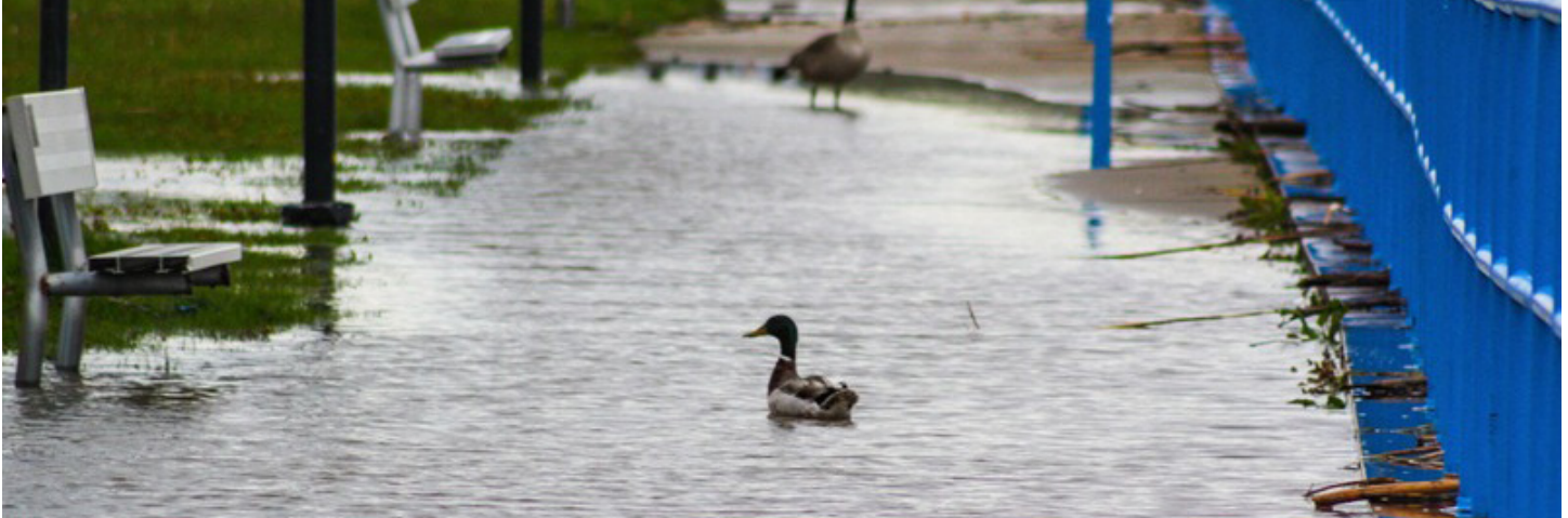
Bay City flooding
