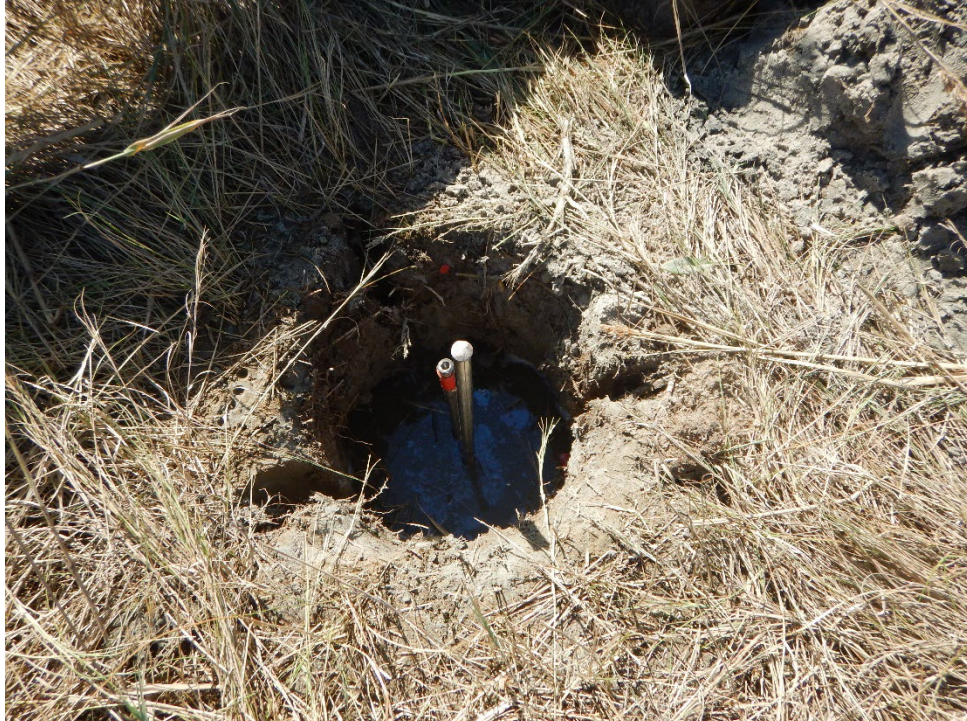
Figure 3: Rod installed into ground before installation of cement-filled PVC collar.
