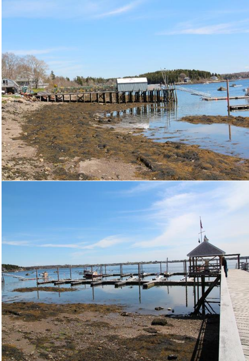
Figure CS3-5. The marina at Basin Point. The equipment and offices (left photo) and slips and moorings (right photo) represent a significant community asset that could be cut off from the town of Harpswell if Basin Point Road floods.
