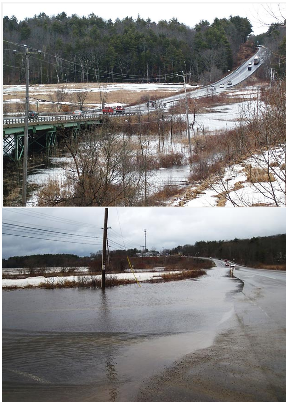
Figure CS2-3. High river flows, an offshore storm, and spring tides in March 2018 combined to cause an extreme high tide that flooded U.S. Route 1 and George Wright Road. The top image shows the area from the west, as cars avoid the water that covers half of U.S. Route 1. The bottom image shows the area from the east, highlighting the flooding on U.S. Route 1 and showing water completely covering George Wright Road to the south.
