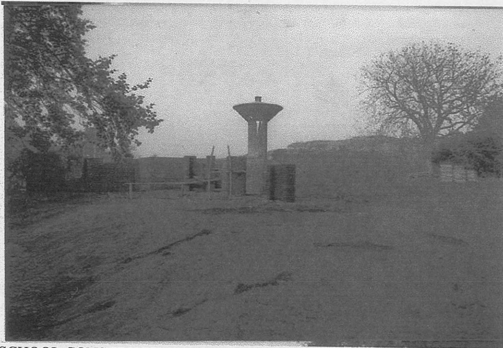
SCHOOL CONSTRUCTION IN PROGRESS. GENEROUSLY SUPPORTED BY CARE FOR THE WILD, UK ; MICHAEL JACKSON, UK, VERA AND SPENCER HODGE, MONACO, KIA MOTORS, SWITZERLAND; SAS SINGAPORE; TIGER ACTION FUND, USA.
